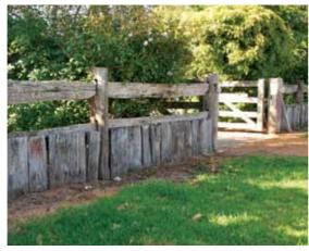
A three-rail jarrah split rail fence near Pemberton, WA (left), and a hybrid split rail/paling fence at Perup, WA (right).
